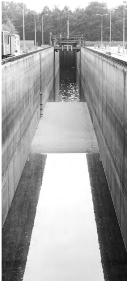
The 230 m-long Delta flume allows waves and sediment transport to be studied at full scale
